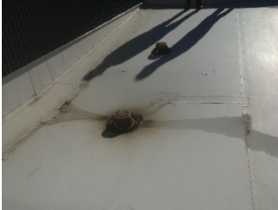
Roof of Crested Butte Community School
