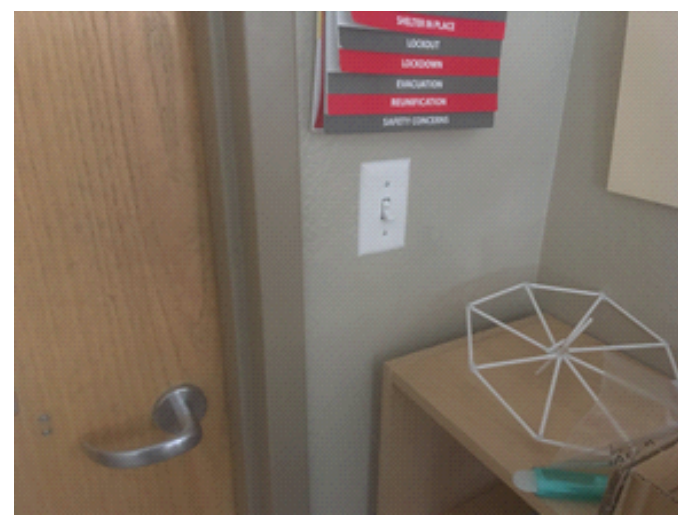
Provide occupancy sensor light switches
